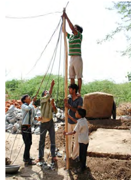
Powerline installation in Rajasthan, India Photo Credit: Gram Power
